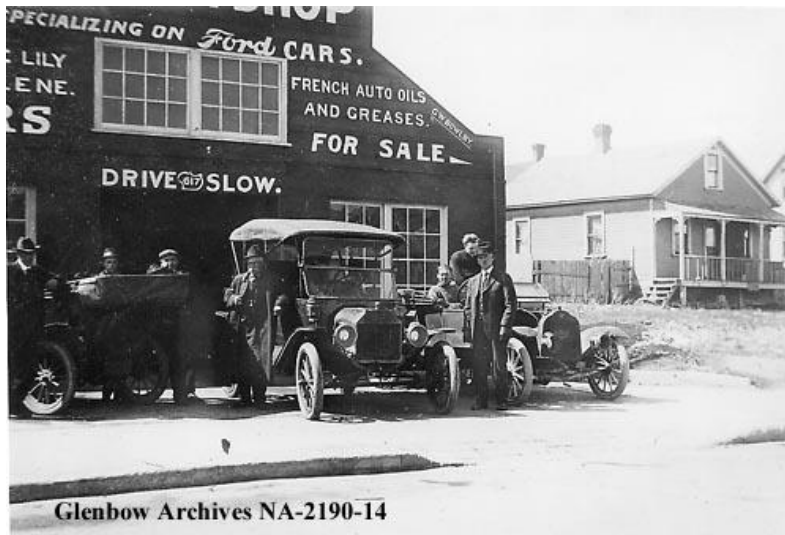
Universal Repair Shop, 1913 (617 7 th Ave SE)
